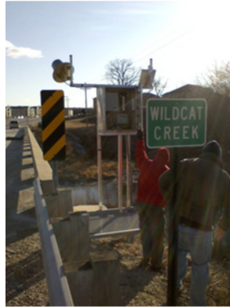
FIGURE 32. WILDCAT CREEK FLOOD STRUCTURE.
