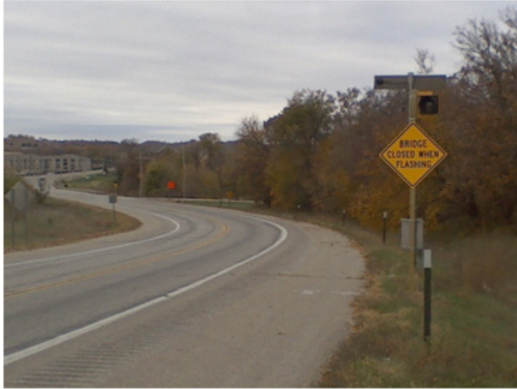
FIGURE 30. BRIDGE WARNING LIGHTS ON WILDCAT CREEK.
