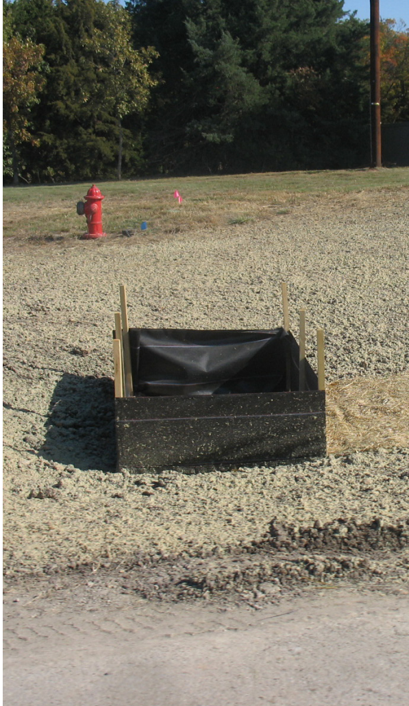
FIGURE 33. PHOTO OF SILT FENCE.
