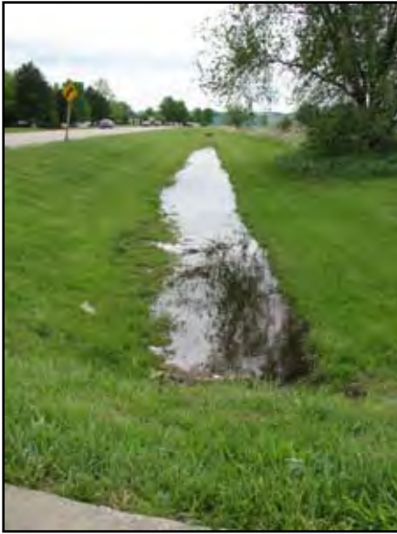
Figure 3.2.3: Looking South along Hayes Drive at D103
