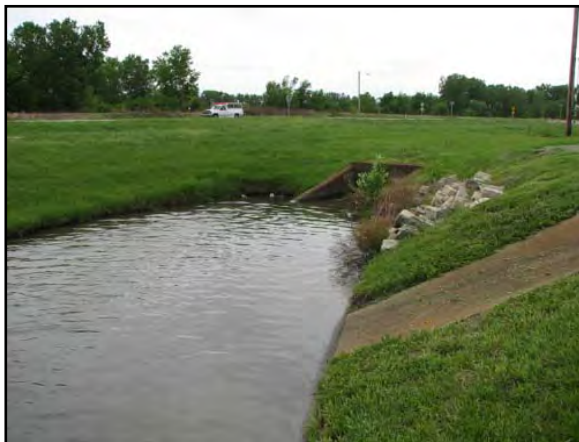
Figure 3.6.5: Looking South at D516 and Entrance to P541 South of Jon Murdock
