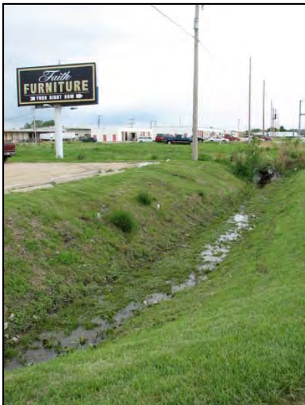
Figure 3.3.9: Looking East along McCall Road at D220
