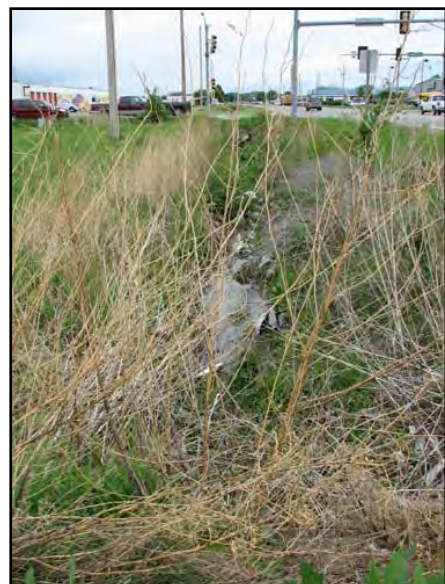
Figure 3.3.8: Looking East along McCall Road at D219
