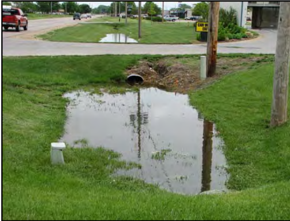
Figure 3.3.3: Looking East along McCall Road at small ditch between P240 and P241
