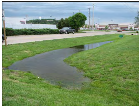
Figure 3.5.2: Looking Northwest along Hayes Drive at D403
