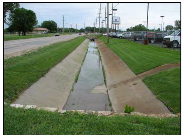
Figure 3.6.2: Looking E along McCall Rd at D513
