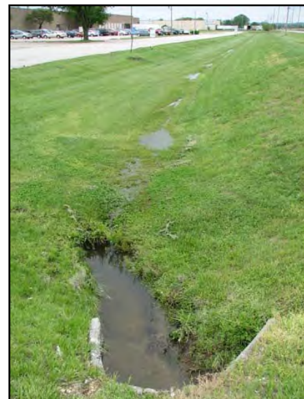
Figure 3.6.8: Looking North on Kretschmer Drive at D507
