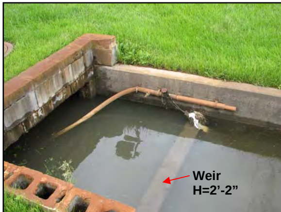
Figure 3.6.7: Closer view of weir in P543 Note water level \pm 6 " above weir
