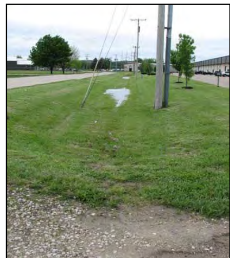
Figure 3.6.16: Looking South along Levee Drive at D518
