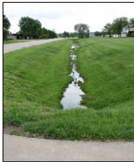
Figure 3.2.2: Looking South along Hayes Drive at D112
