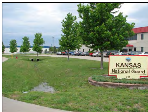
Figure 3.4.4: Looking Northwest along Levee Drive at D310
