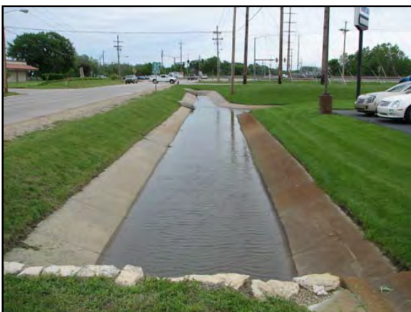
Figure 3.6.3: Looking E along McCall Rd at D514
