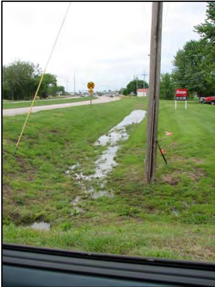
Figure 3.6.17: Looking Southwest along HWY 24 at D522
