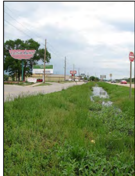
Figure 3.6.18: Looking East along HWY 24 at D534
