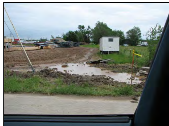
Figure 3.6.10: Looking East at GTM Expansion from Carlson Street
