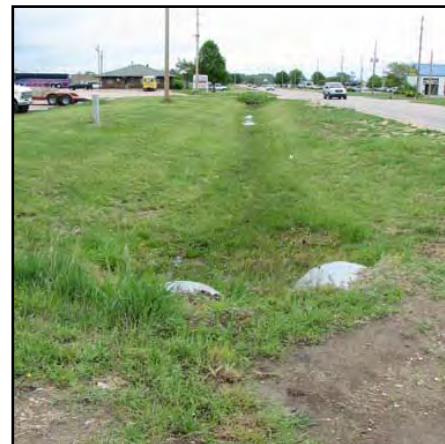
Figure 3.3.6: Looking East along McCall Road at D217
