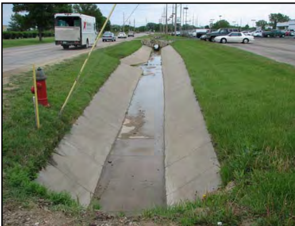
Figure 3.6.1: Looking E along McCall Rd at D512
